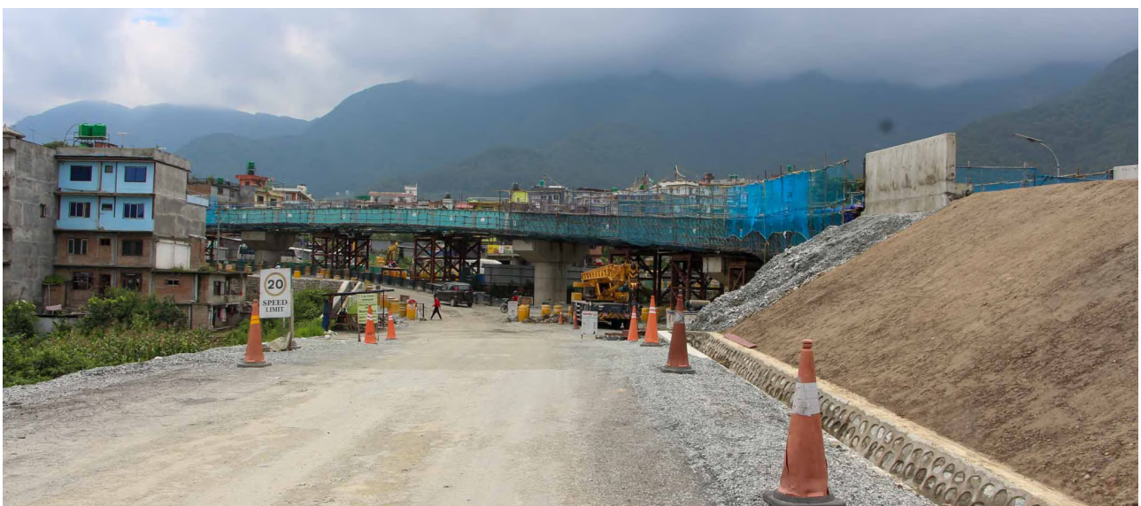
Flyover under construction phase © UN-Habitat, 2024
